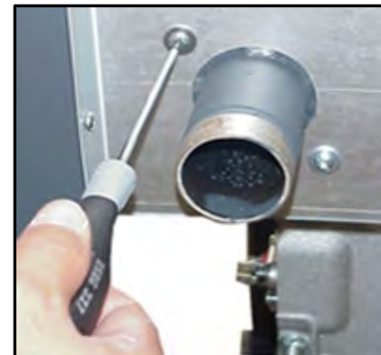
Figure 7: Removing Intake Filters
